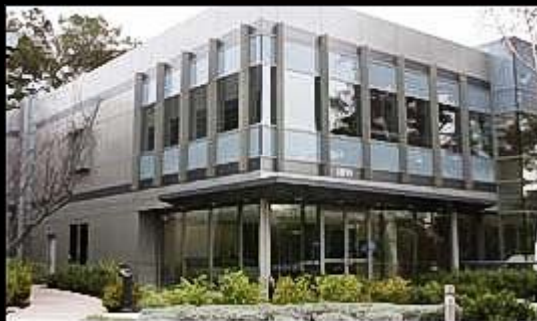
Corning West Technology Center Silicon Valley, California
